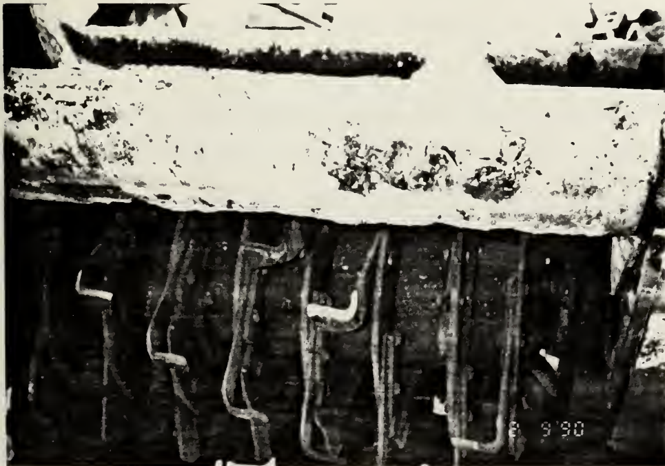
Figure 2.11 Soil Stabilizer Mixing Tines
